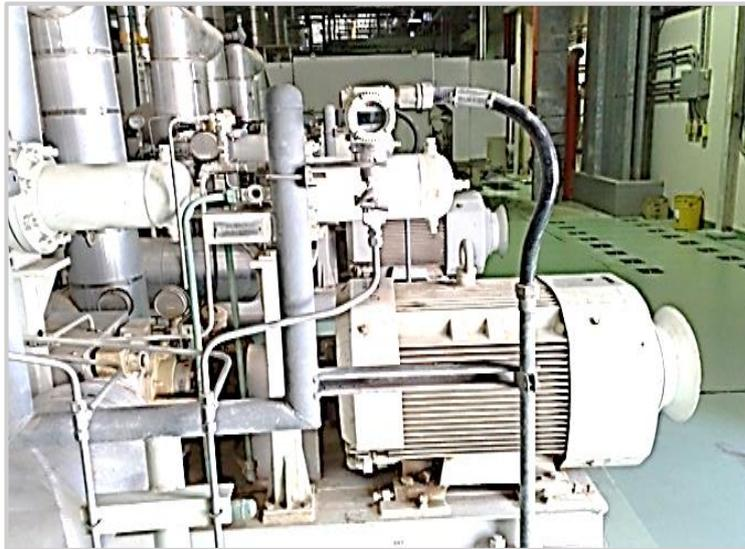
Figure 2. X1 location: Low Pressure Feed Pump (STU3).
